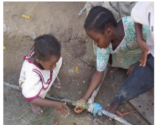
Multiple leakages along the damaged water network
